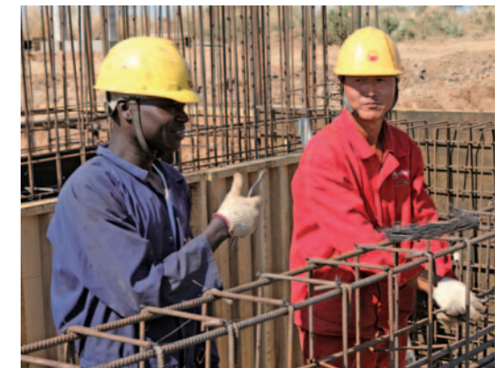
Gas pipeline in Tanzania
