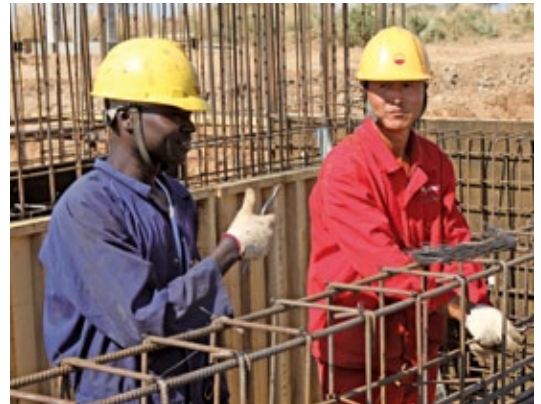
Gas pipeline in Tanzania
