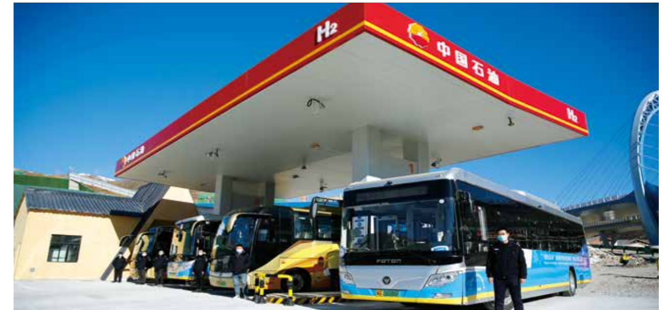
Hydrogen refueling station serving the 2022 Winter Olympics
