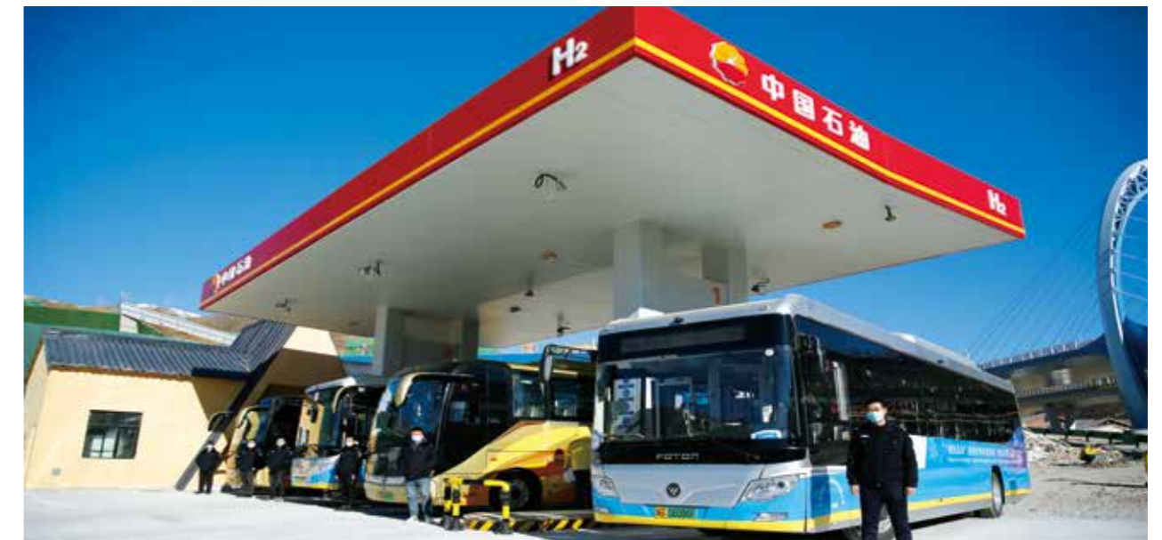
Hydrogen refueling station serving the 2022 Winter Olympics
