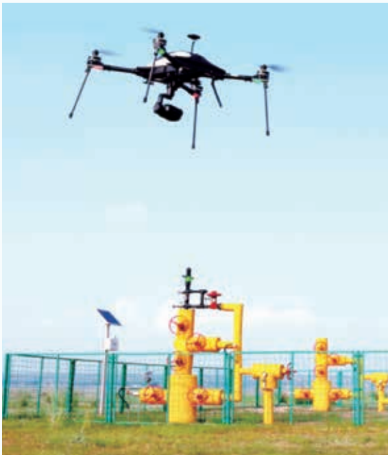
Routing inspection by drones at Changqing
