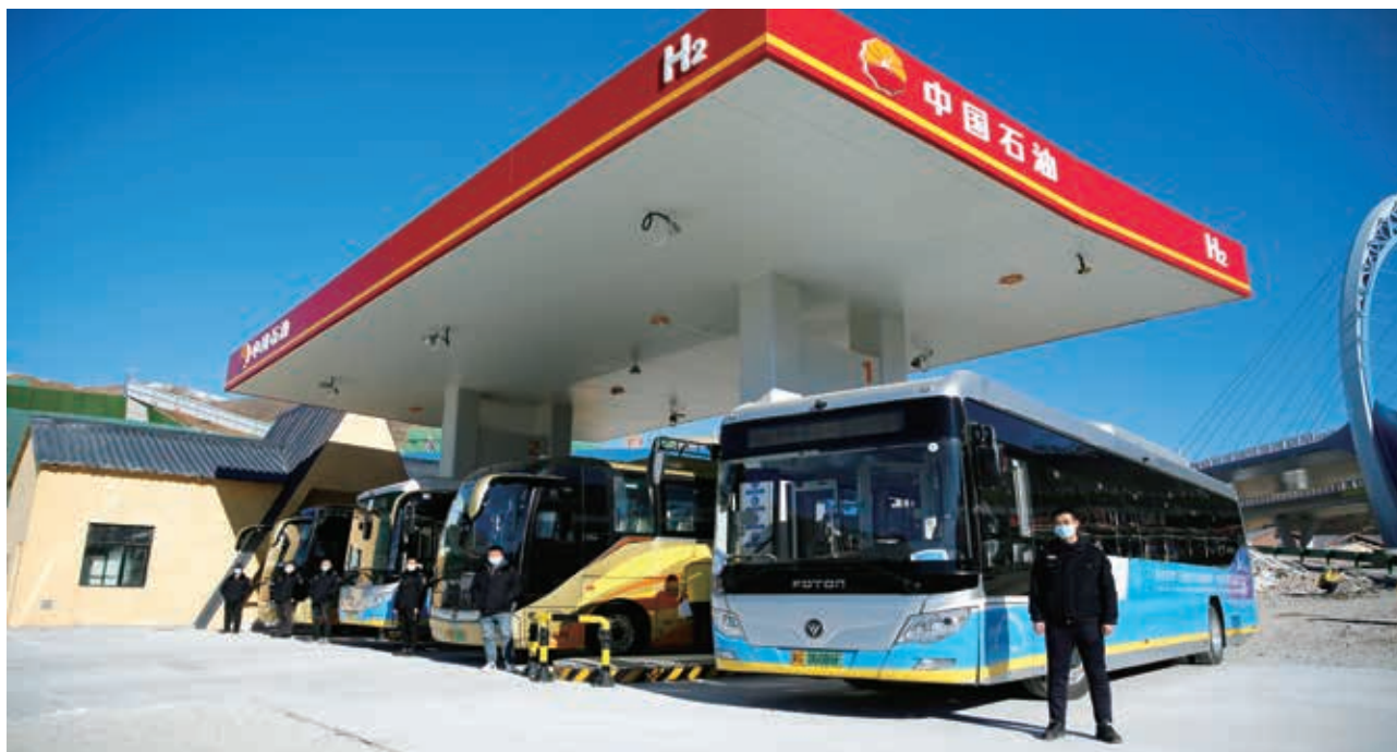
A CNPC hydrogen refueling station
