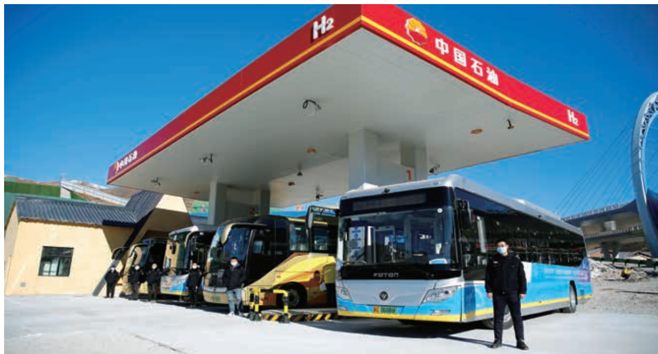
A CNPC hydrogen refueling station
